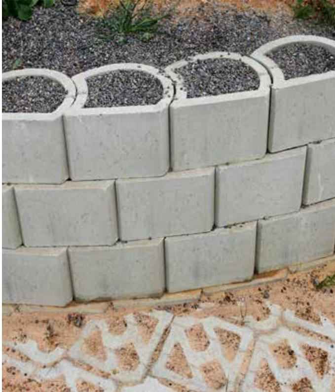
Sides built using Terraforce L11 Smooth blocks
