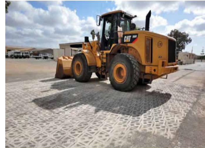
Blocks are underlain with 100mm compacted sand, over sub base of rubble
