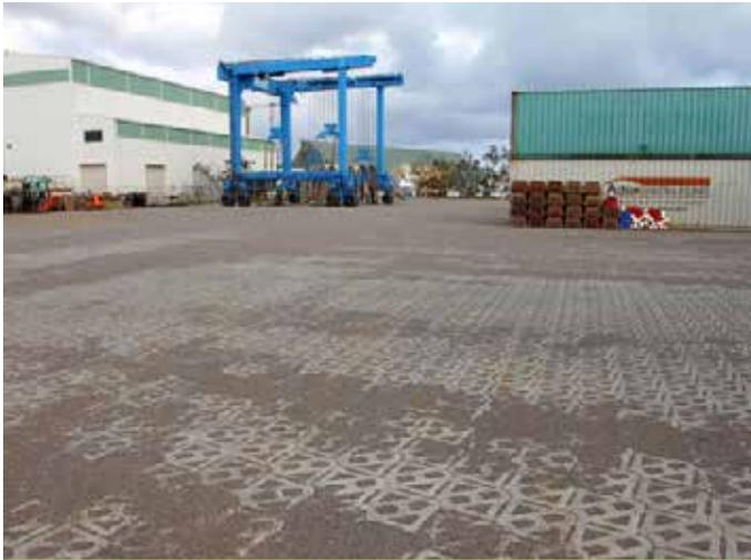
Permeable paving for a boat lifter facility
