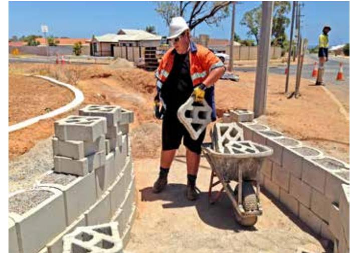
Storm water channel, using the interlocking, permeable Terracrete blocks
