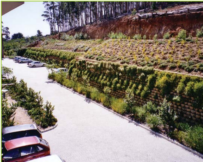
COMPOSITE RETAINING WITH TERRACING AND PLANT COVER
