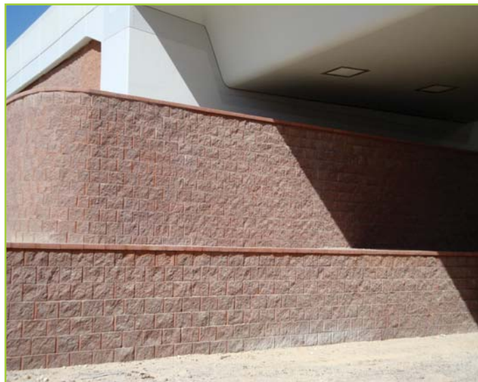
RETAINING WALL AT INTERCHANGE IN DUBAI
